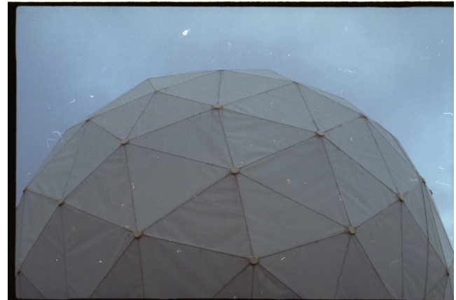
SvalSat satellite ground station, Platåberget, Svalbard 2025
