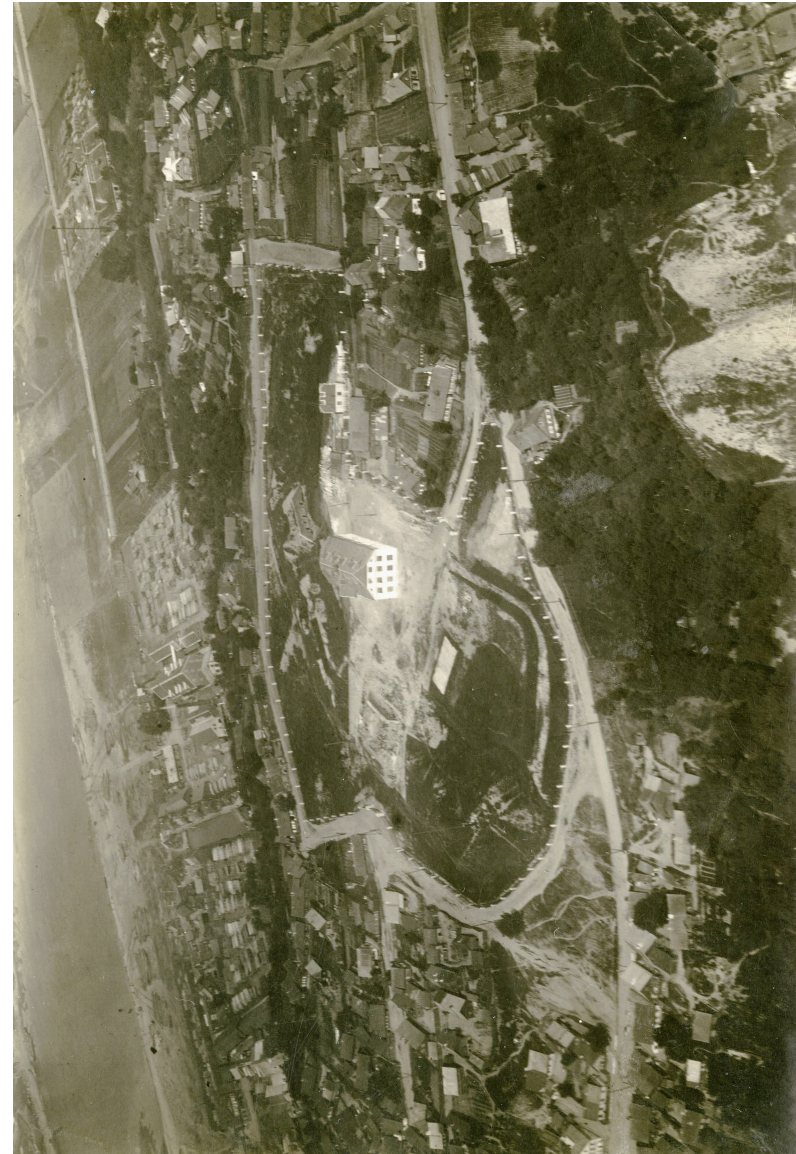
Owl Hill, construction of Kaunas Art School, 1922–1923. Courtesy of Lithuanian Aviation Museum.
