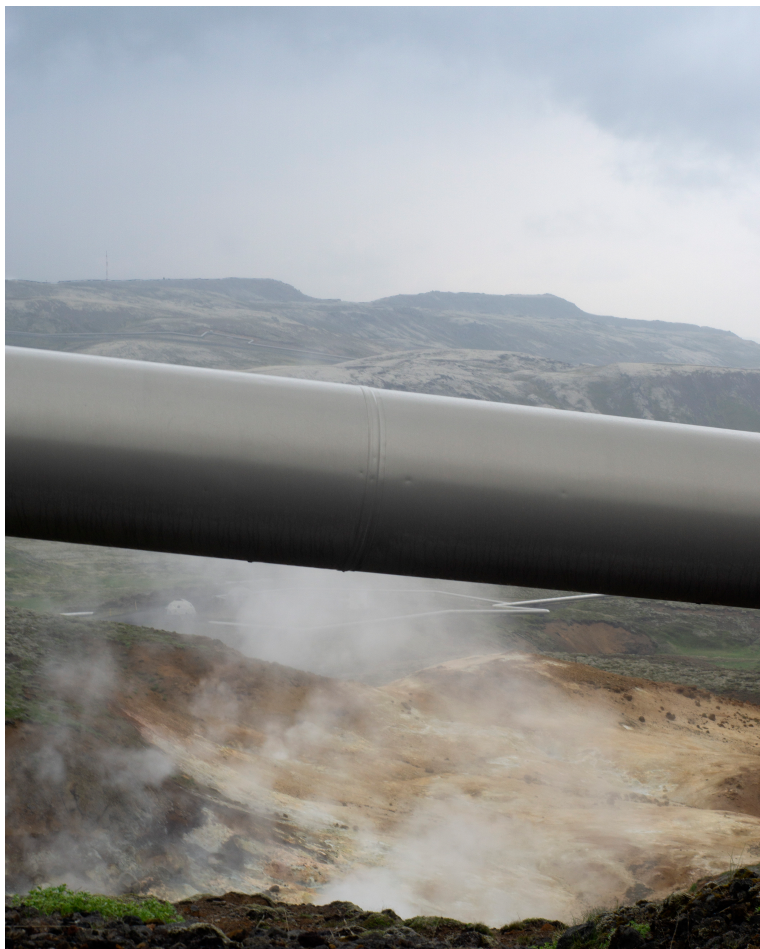
Fig. 1.: Untitled, pipeline near the Nesjavallavirkjun geothermal power plant, digital photograph, 2024
