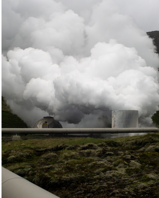
Fig. 5.: Untitled, borehole and pipes near Nesjavallavir geothermal power plant, digital photograph, 2024
